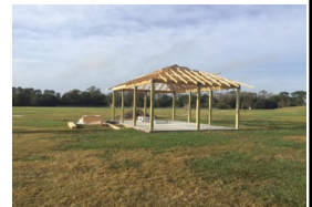
PAVILION IN PROGRESS
